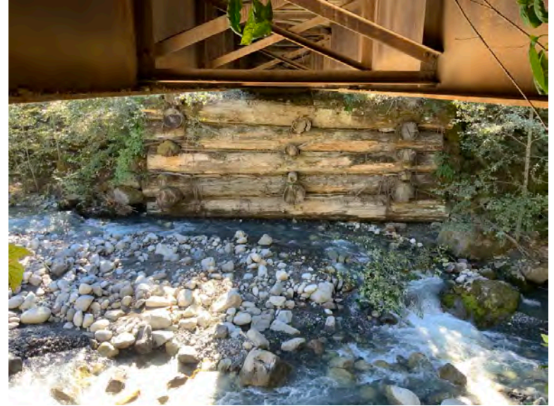
Left Bank Abutment when facing downstream
