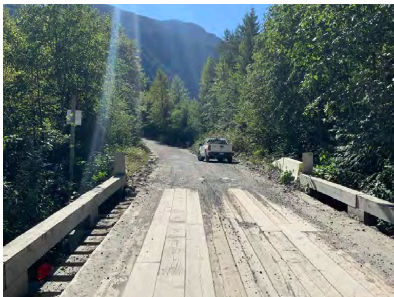
Approach from Left Bank when facing downstream
