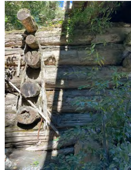
Right Bank Abutment when facing downstream
